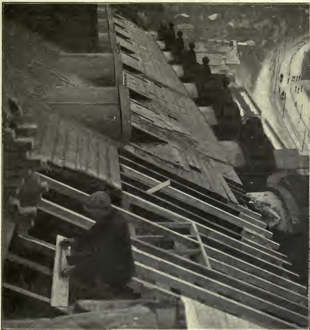
SCARBOROUGH: ROOF OF THE GRAND HOTEL, ["Times" Photograph. Which was badly damaged at both ends.
