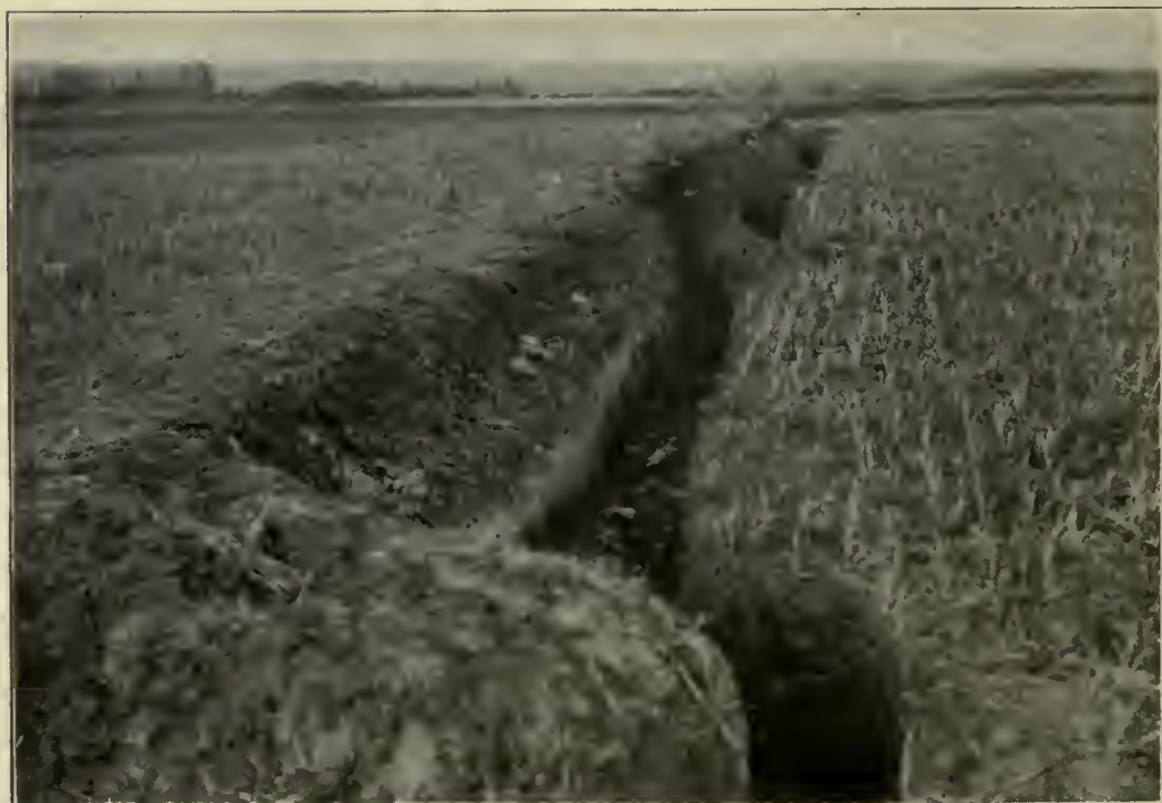
GERMAN TRENCH IN PRACTICE, Showing the traverses.
