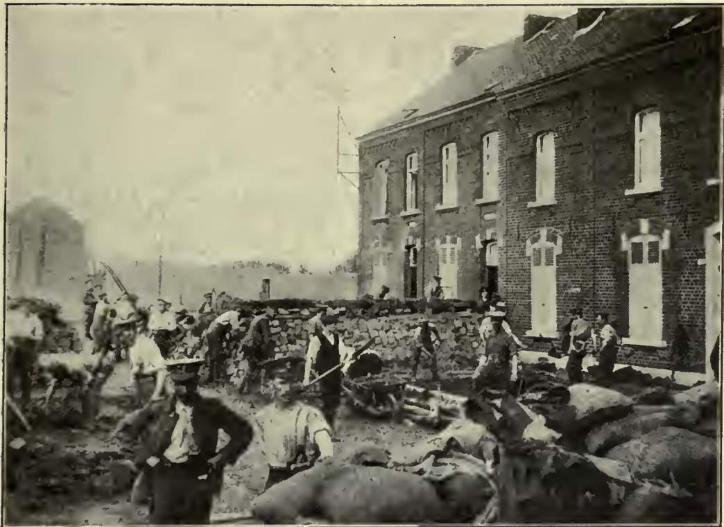
BRITISH SOLDIERS ERECTING BARRICADE ON THE OUTSKIRTS OF A FRENCH TOWN.
