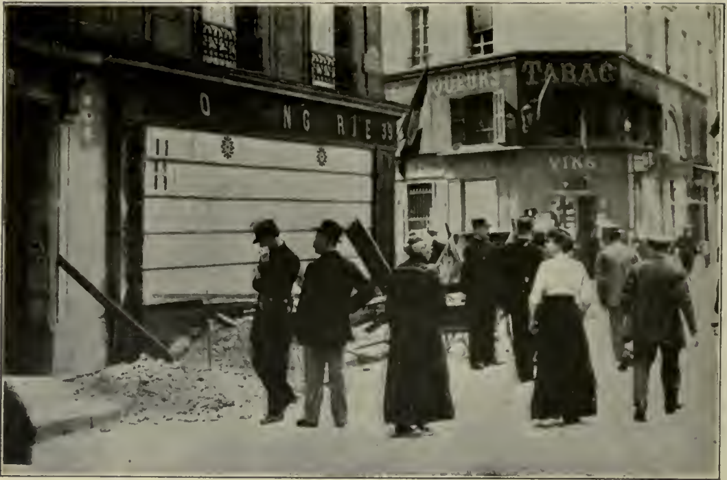
RUE DES VINAIGRIERS. Damage done by bomb from German aeroplane.
