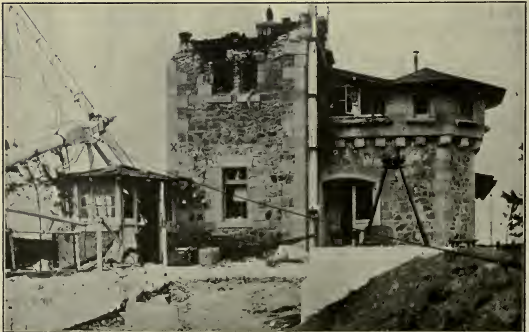
TSING-TAU WIRELESS STATION DESTROYED.
