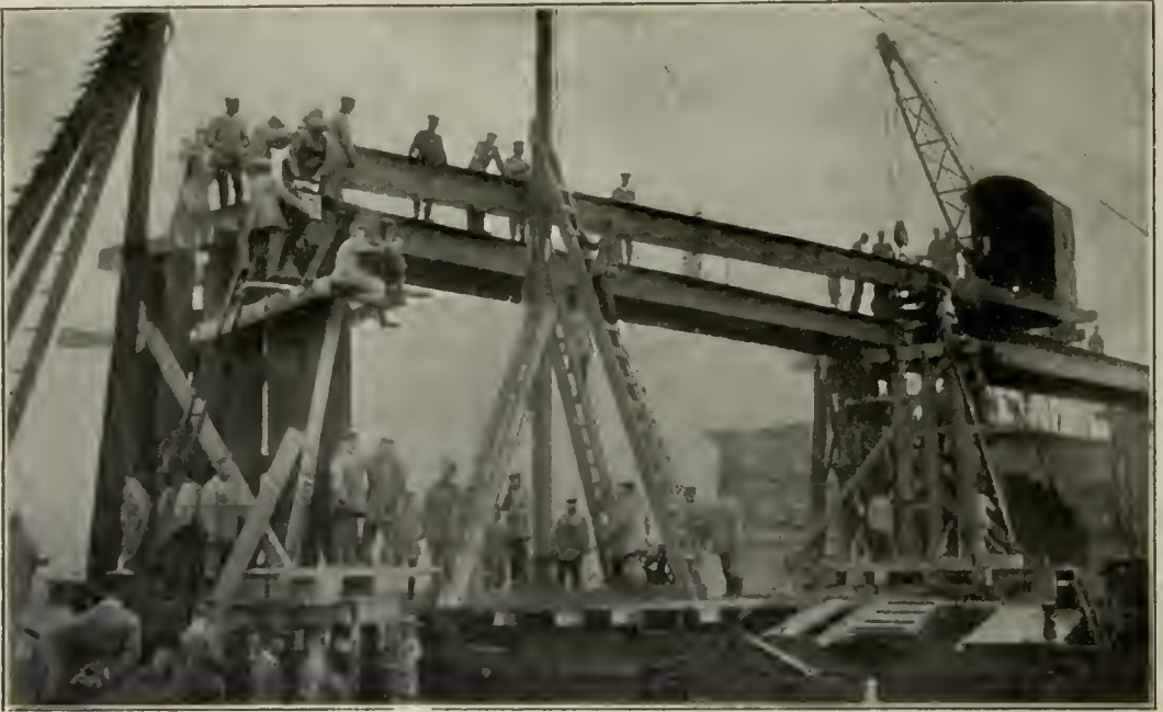
GERMANS ERECTING AN IRON BRIDGE IN PLACE OF THE ONE IN THE BACKGROUND, WHICH WAS DESTROYED.
