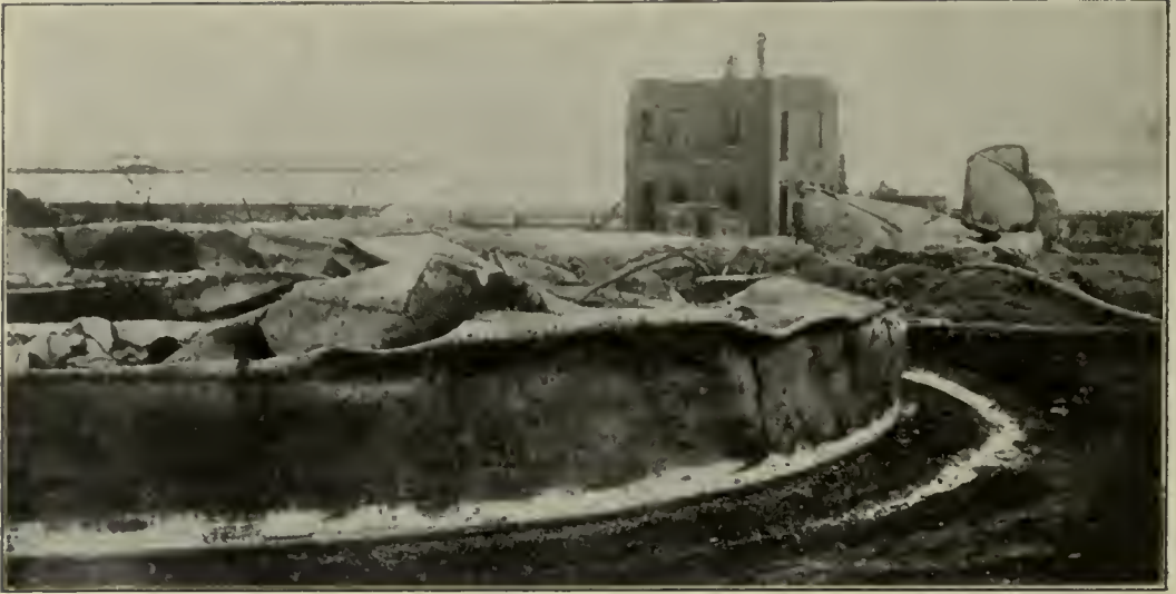
OIL TANKS DESTROYED AT TSING-TAU.
