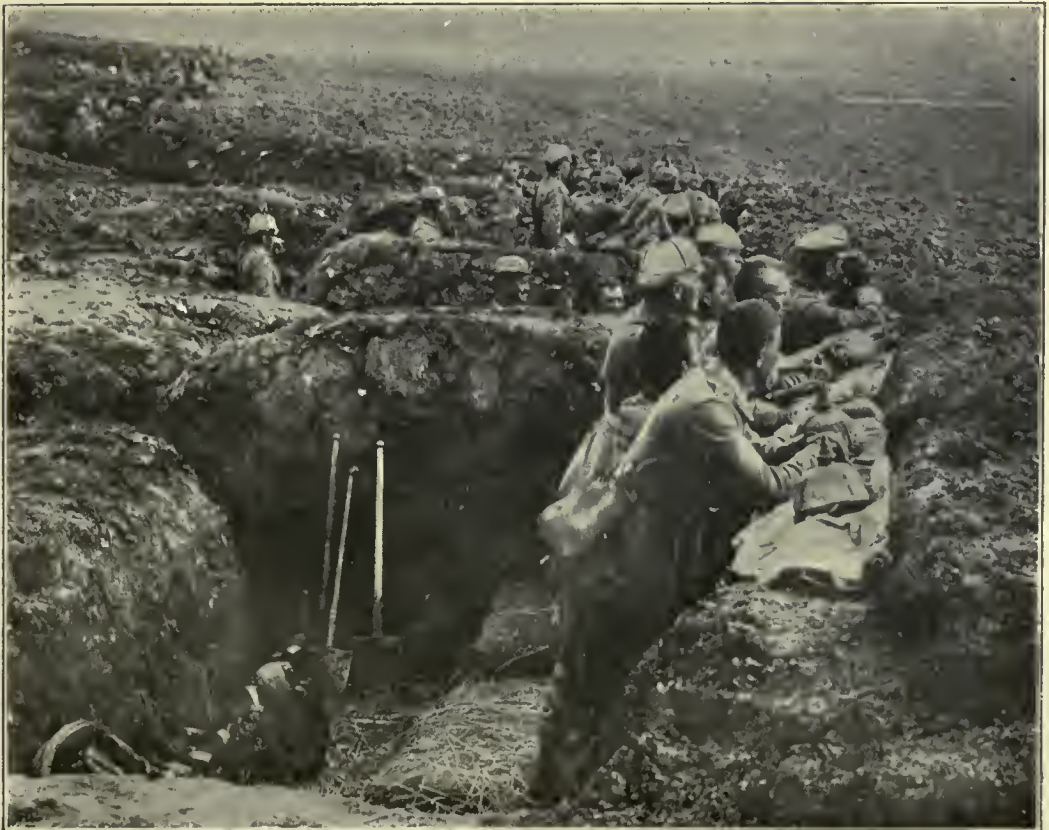
GERMAN TRENCH, SHOWING THE ZIGZAG FORMATION AND TRAVERSES.
